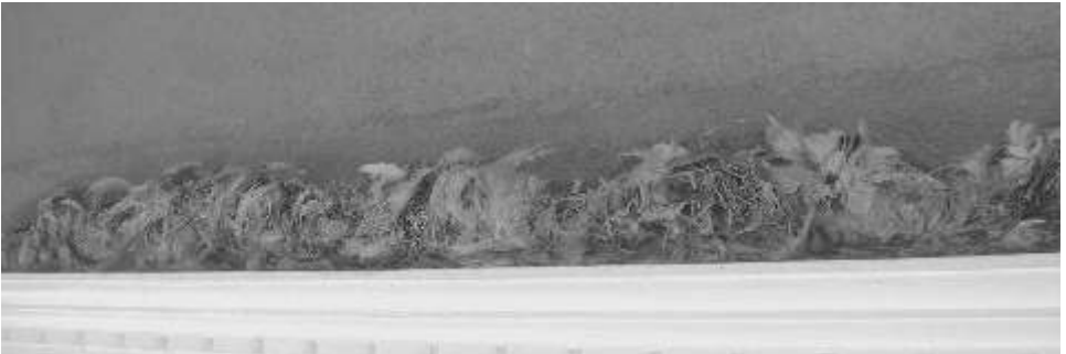
Under all these feathers and other debris are spikes - instead of keeping birds away they accumulate nesting material and make ideal nesting spots.
