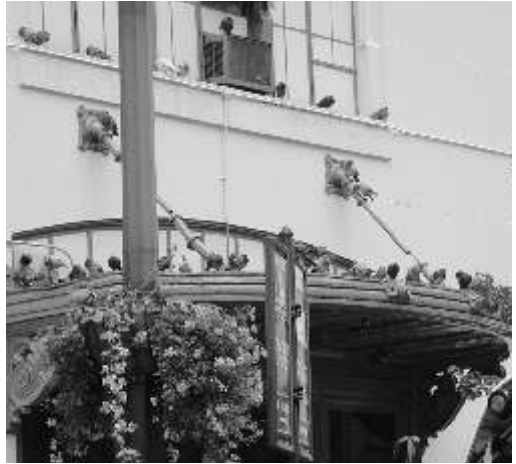
It's actually unsafe to enter this building without an umbrella!
